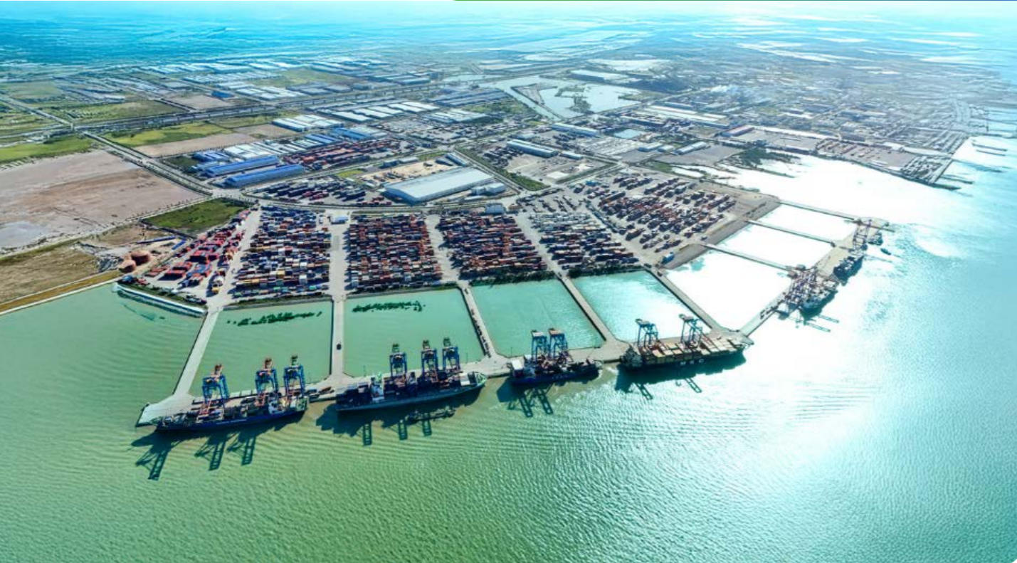
Nam Dinh Vu Port Phase 3 officially commenced operations in October 2025
