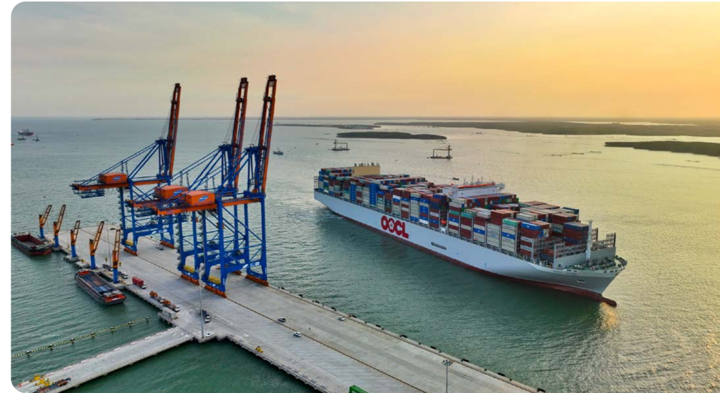
Gemalink Port: The only port in the region with the infrastructure and technology to accommodate the world's largest mega-container vessels.
