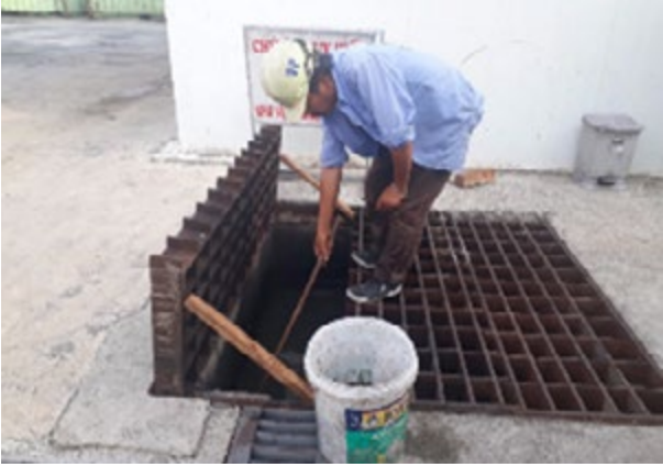
Cleaning, dredging, utilizing access holes to collect water
